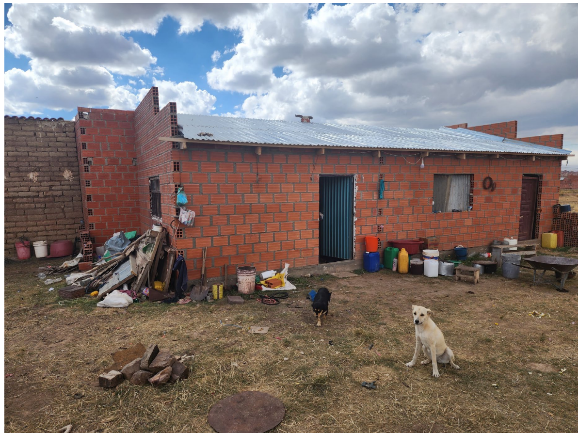
This is Flora's house where we took the sensor box to be tested during cooking hours. There was no chimney at this house. The ventilation was a crack between the roof and the outside wall the roof attached to.
